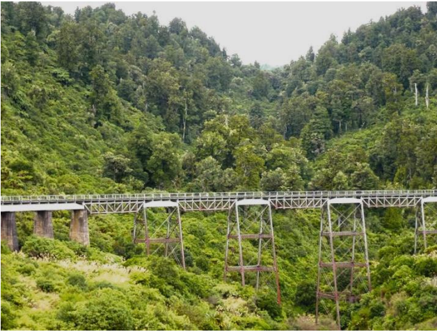
Fig. 8: Restored Hapawhenua Viaduct, 27 March. Photo: Richard Hursthouse.
