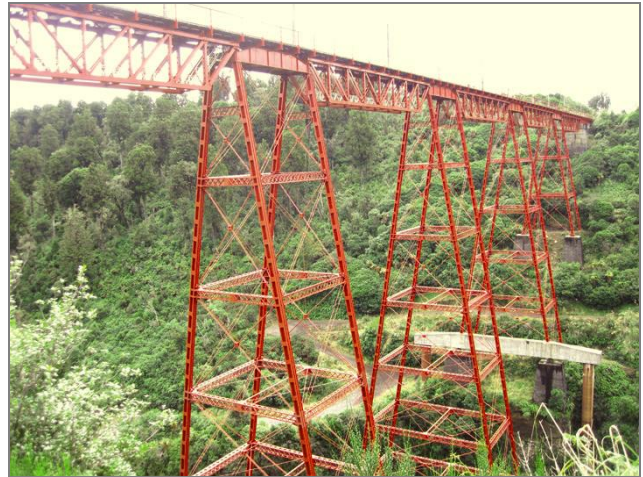
Fig. 5: Makatote Viaduct, 25 March.
