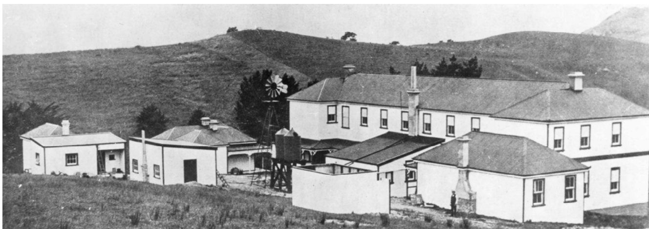
Fig. 4. The new accommodation block for 100 men ( Weekly News Supplement , 24 Nov 1910, p.12) – it burnt down in 1973. Auckland Museum neg, no. C10841.
